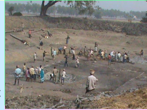
Excavation of ponds Under MGNREGS
